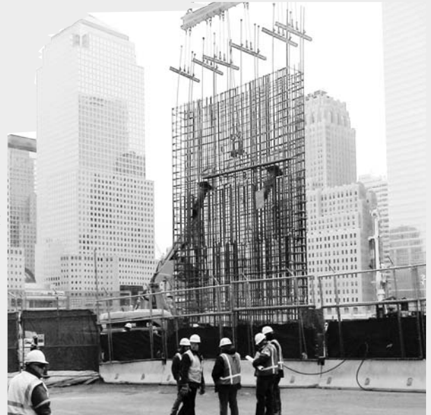
Steel girders of Bathtub being laid into place.
